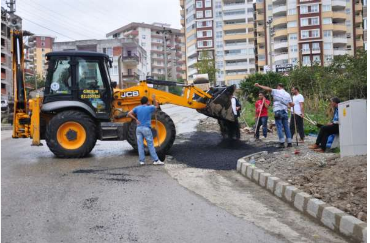
7. AKSU MAHALLESİ PAZAR CADDESİ(2600 mt)
