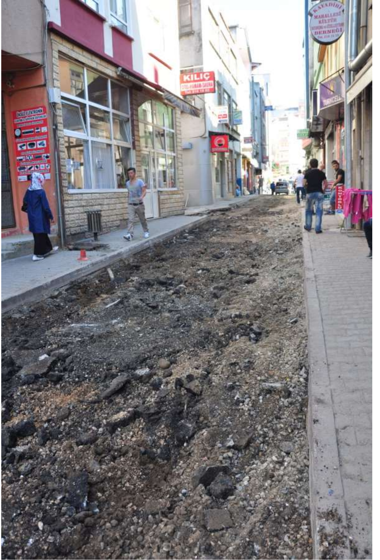
12.OSMANIYE MAHALLESİ HASAN VEHBİ SOKAK PARKE ONARIM
